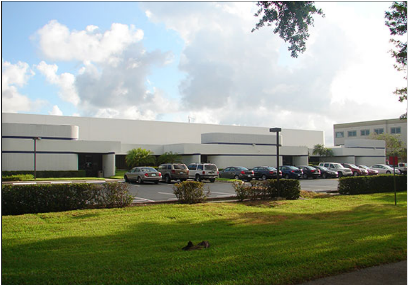
1155 Northwest Broken Sound Parkway, one of seven properties sold to Adler Kawa
