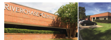
Riverchase Center, Birmingham Alabama
